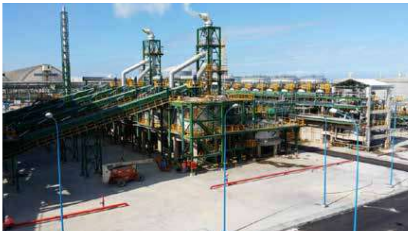
Pic 1: 6,000 tons per day capacity - Sulphur Melting & Filtration plant
